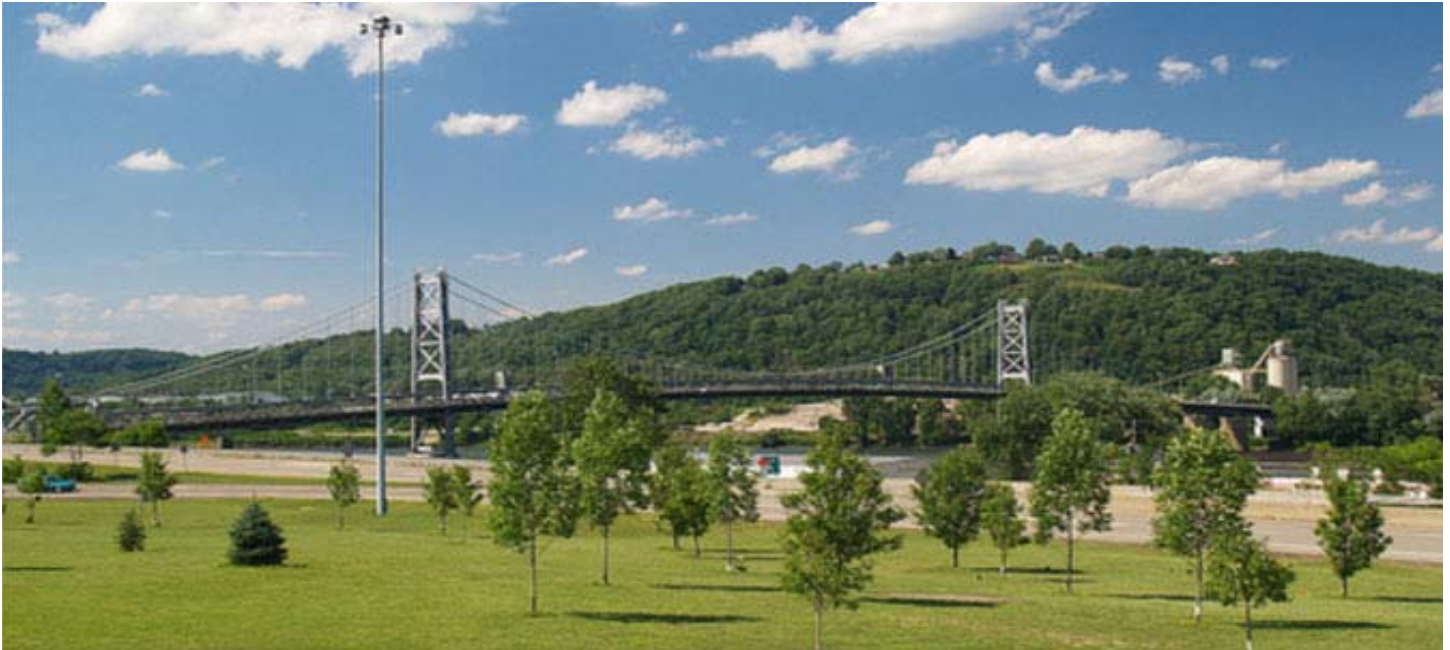
Bridge over the Ohio River at Steubenville
