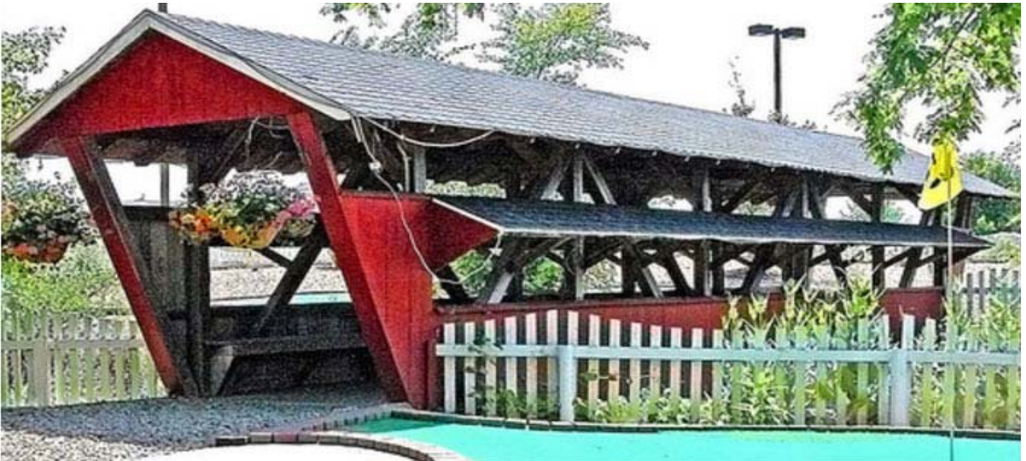
Hoagland Covered Bridge, east of Hillsboro
