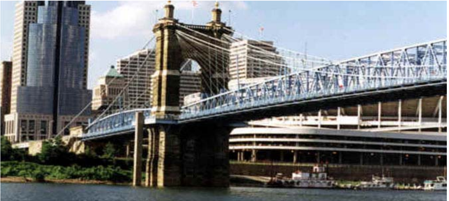
John A. Roebling Suspension Bridge, Cincinnati
